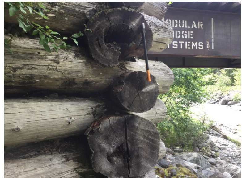
Typical face log condition at ends
