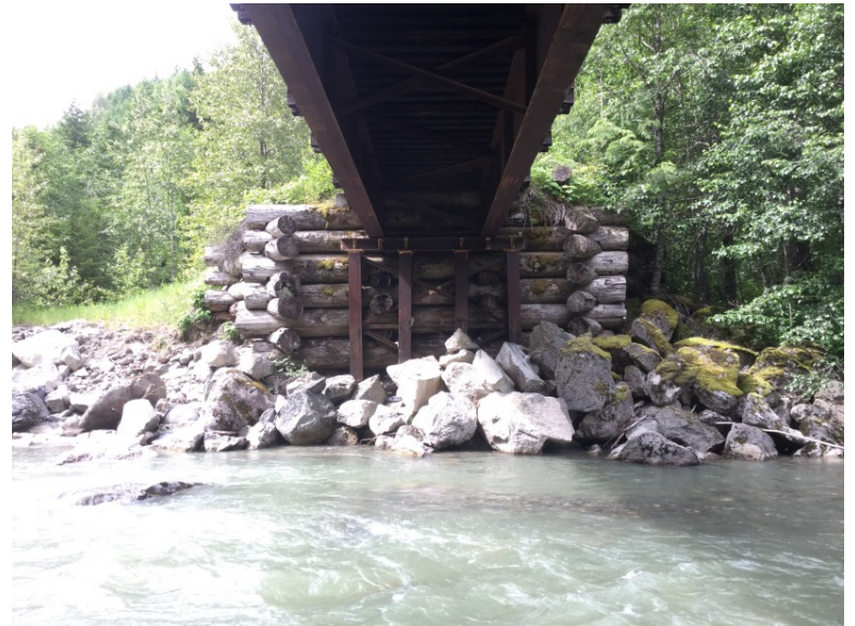
Left Bank Abutment when facing downstream
