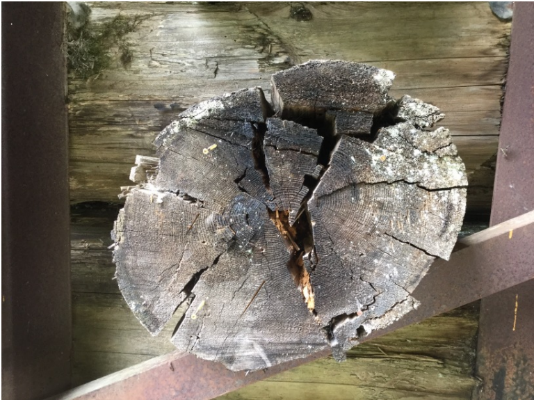
Tieback condition at right bank
