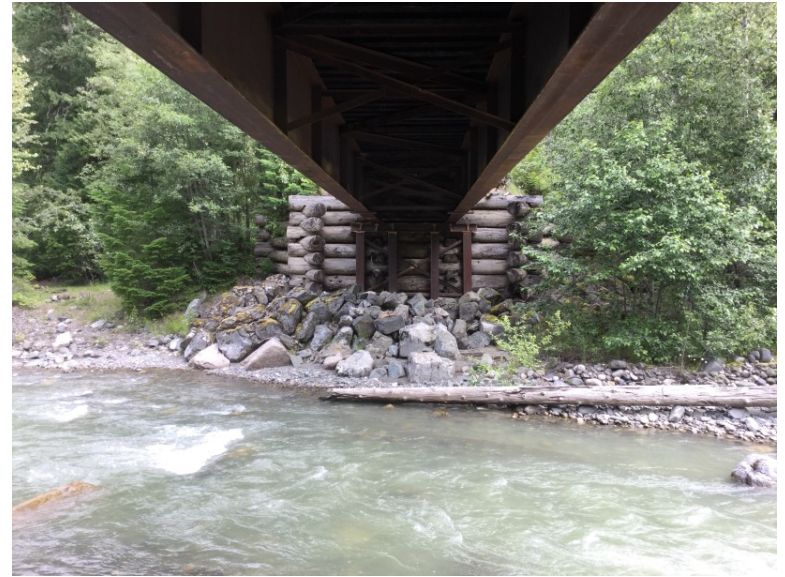
Right Bank Abutment when facing downstream
