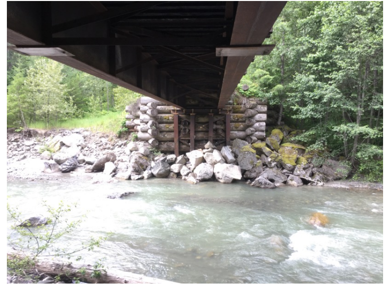
Left Bank Abutment when facing downstream
